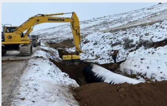
South Branch Canal piping project, January 2024
