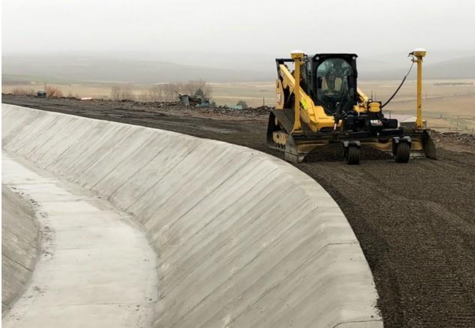
North Branch Canal lining project, Winter 2023
